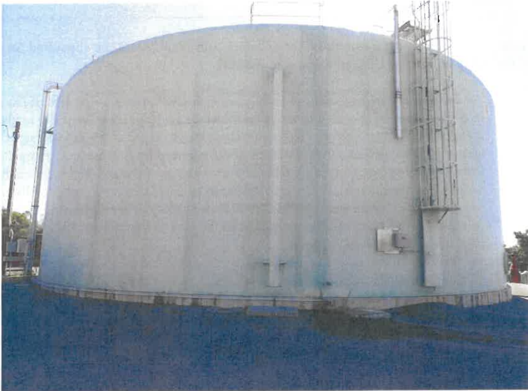
Overall view of the tank.
