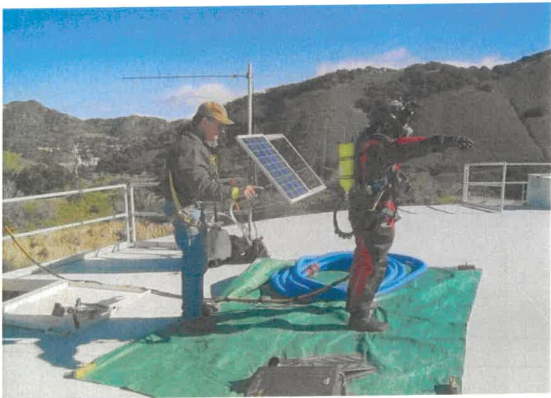
Diver and equipment are disinfected with the chlorine solution just prior to entry. This procedure is pursuant to AWWA disinfection standards for potable water diving (stock photo).
